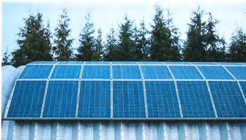
Hakai Energy Solutions found a way to install solar panels on the curved roof of Alert Bay's public works building. Photo by Sean Fenzl.
